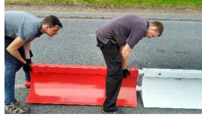
2. Slot together, use pin as handle as needed
