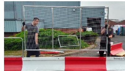
Insert panel pins into min 3 aligned Fortis or Fortis Crash as shown, ensuring panel overlaps barriers
