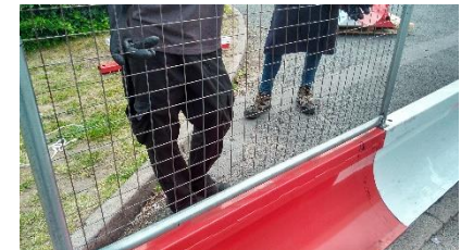
Insert panel pins into min 3 aligned Fortis or Fortis Crash as shown, ensuring panel overlaps barriers
