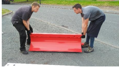
1. Lift into position (2 x man lift)
