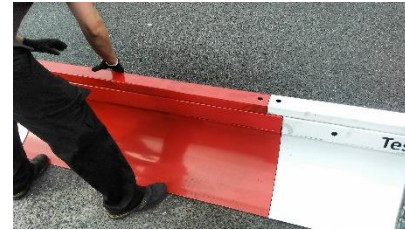
3. Ensure brace overlaps barriers
