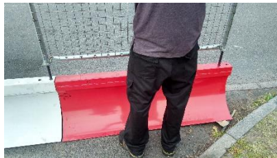
Insert panel pins into aligned Fortis or Fortis Crash as shown, ensuring panel overlaps barriers
